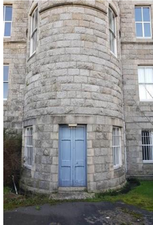
Plate 24: Bowed bay with panelled double doors at rear of Tabor House
