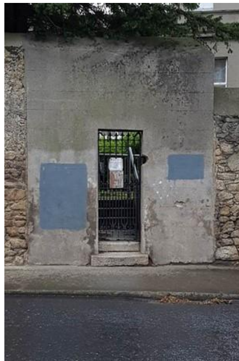
Plate 69: Side gate on Sandford Road, no longer in use, cut granite step and rendered walls
