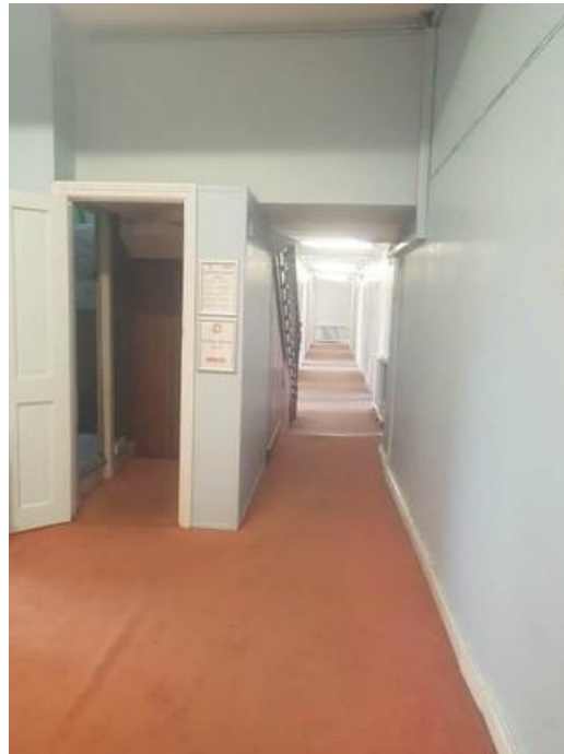
Plate 117: Central hall at 2 nd floor level linking to rear extension block. Note water tank room to lhs of image which extends up into roof void
