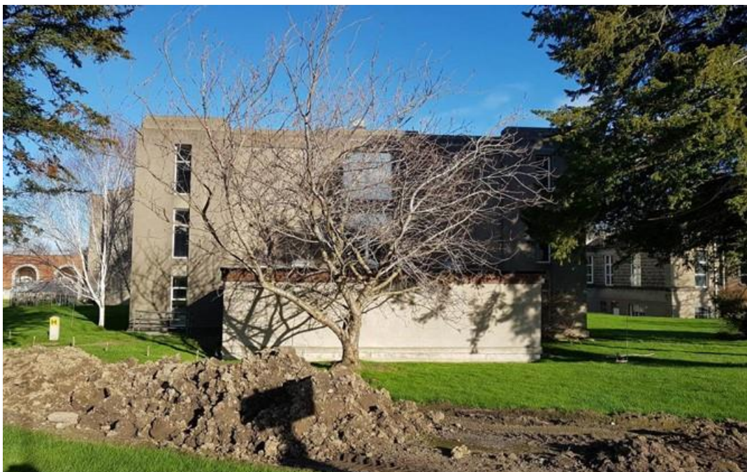
Plate 48: South-west gable of archive with 1970's single storey extension in foreground
