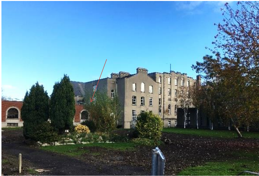
Plate 61: Southwest view of the rear extension with the red brick, link building (principally outside the applicant boundary) in view
