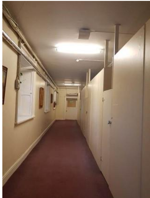
Plate 189: Alternative basement corridor to fire door
