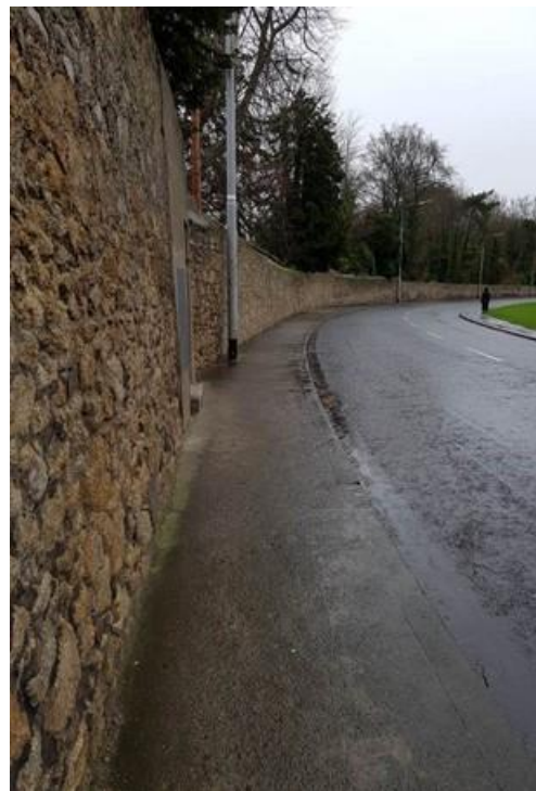
Plate 76: Curve of wall looking down Milltown Road, with pedestrian gate in centre
