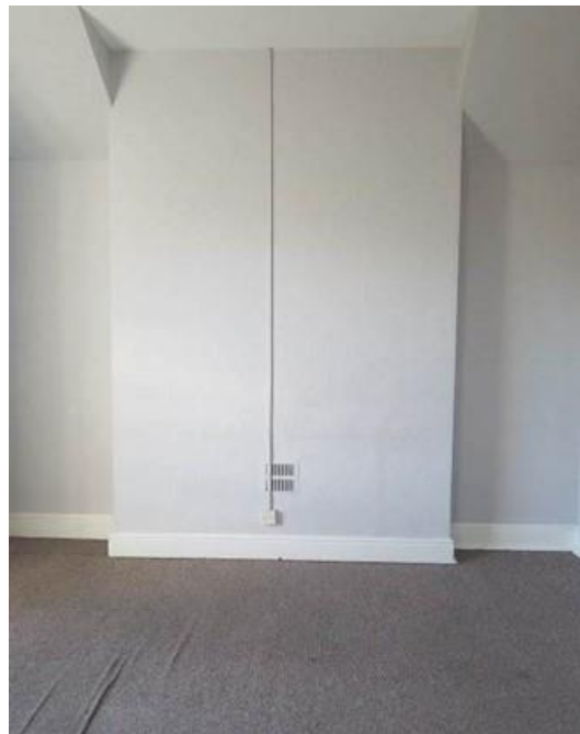
Plate 199: Example of removed chimney piece to typical bedroom
