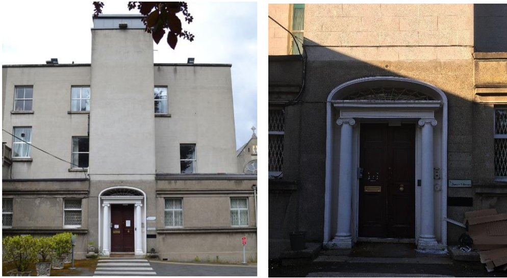
Fig.17/18 Present day configuration of east (front) elevation of Milltown Park, with the vertically extended entrance lobby; vertical extension to south (denoted by higher level windows) and repositioning of first floor windows. Fig.18 shows a detail of the surviving entrance door and fanlight within a much altered context.
