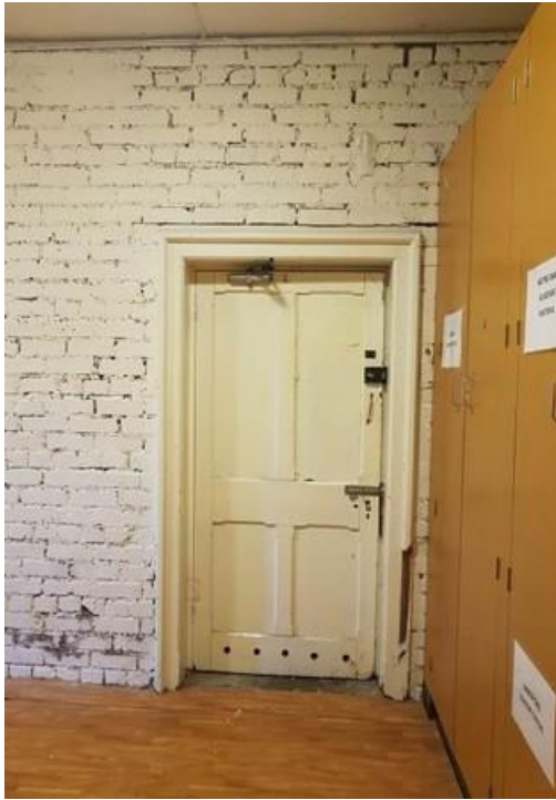
Plate 186: Services area at lower ground floor level with original walls exposed and painted
