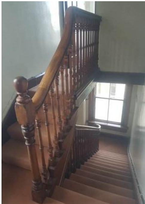
Plate 156: Detail of stair from 2 nd to 1 st floor
