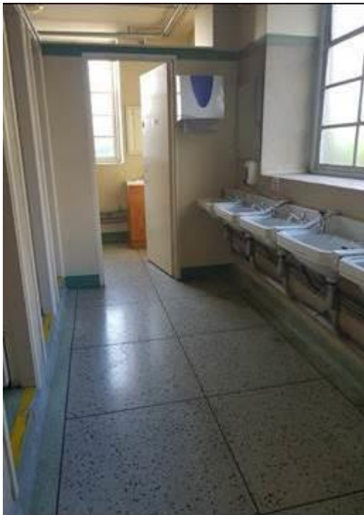
Plate 257: Toilets within the same area
