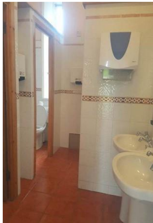
Plate 138: Toilet block within 1 st floor level
