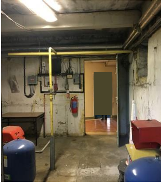
Plate 98: View from plant room towards central corridor
