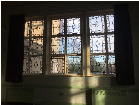
Fig.45 North elevation leaded window
