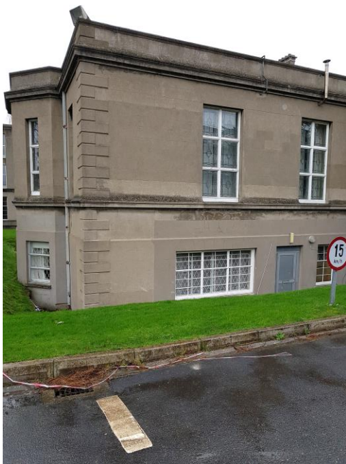
Plate 43: Eastern elevation of Finlay wing
