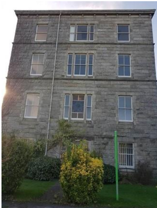
Plate 25: North east gable elevation of Tabor House
