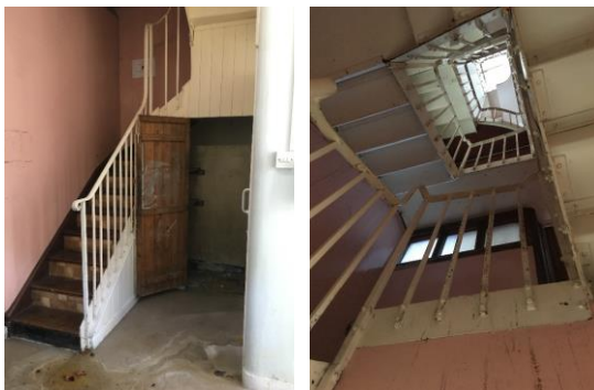
Fig.65 Secondary steel stair of interest
