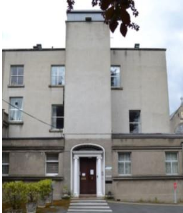
Plate 1: Milltown Park House entrance with some of its many extensions visible
