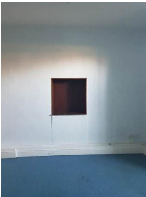
Plate 180: Access to dumb waiter now covered
