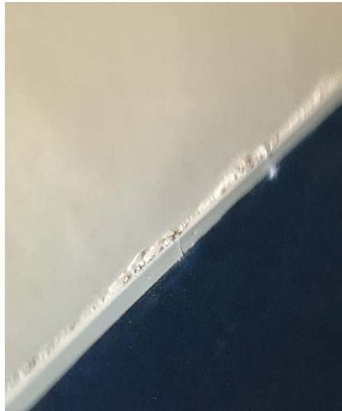
Plate 103: decay of skirting boards within corridor
