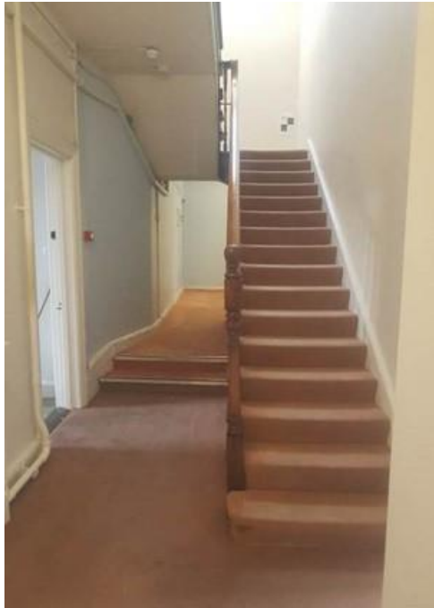
Plate 154: Stair at rear of block
