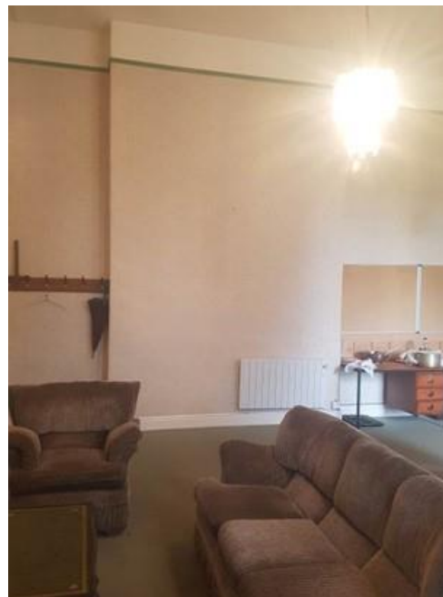
Plate 93: Large chimney breast without fireplace
