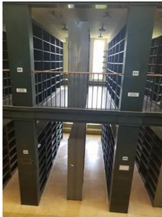
Plate 266: View of the metal structure aligned with custom built bookshelves
