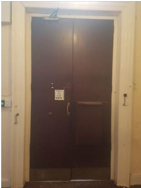
Plate 128: Security door off main block corridor
