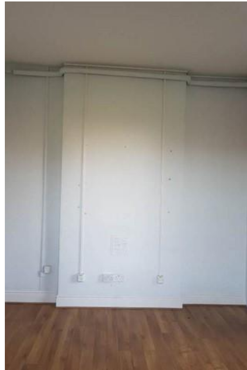
Plate 179: Chimney breast without fireplace
