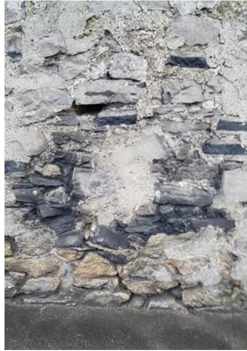
Plate 74: Composition of boundary wall varies, sections of rubble wall have been infilled
