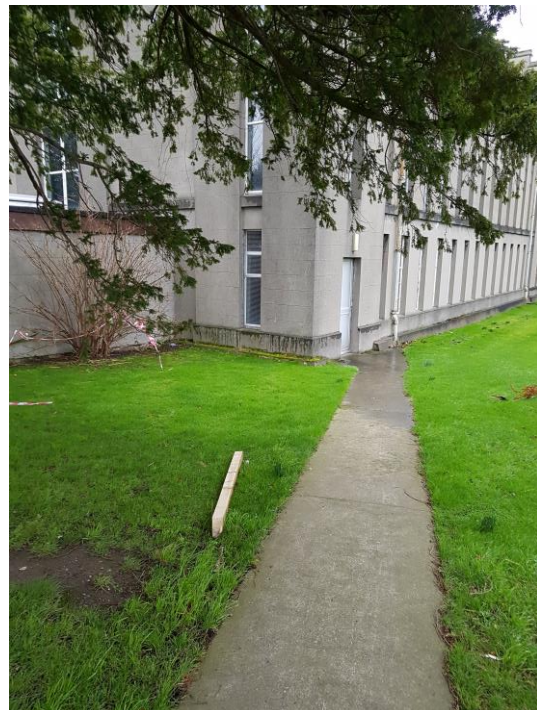
Plate 59: East elevation, gable to south
