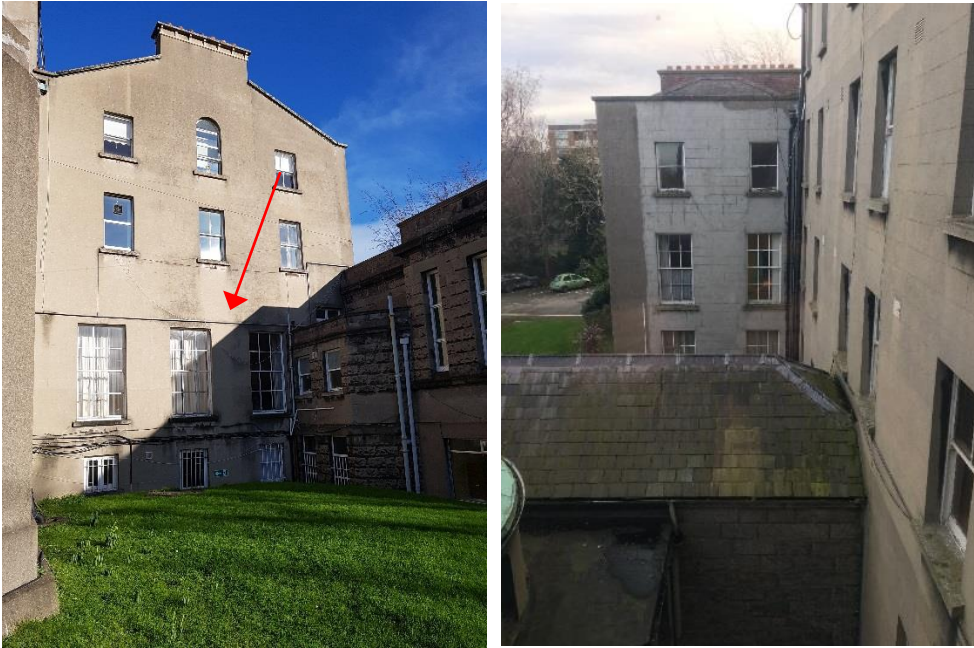
Fig.21 Southern elevation, comprising an extension, with its expressed gable in context with the Finlay Wing and Archive (corner visible). Lower windows are early in origin, with the 6/6 windows attached to a former orangerie, which was vertically extended in the 20 th century.
